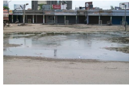
Water logging problem due to poor drainage
