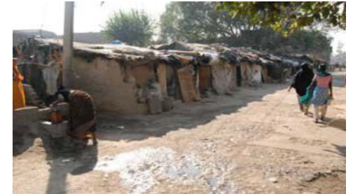
Dilapidated houses / slums at Sangrur
