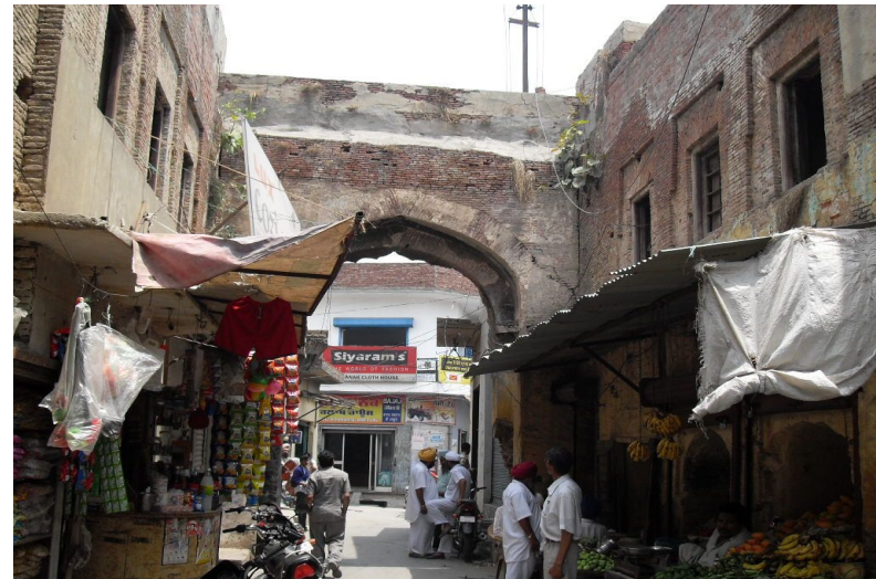
HISTORICAL LAHORI GATE CONVERTED INTO SHOPPING CENTER
