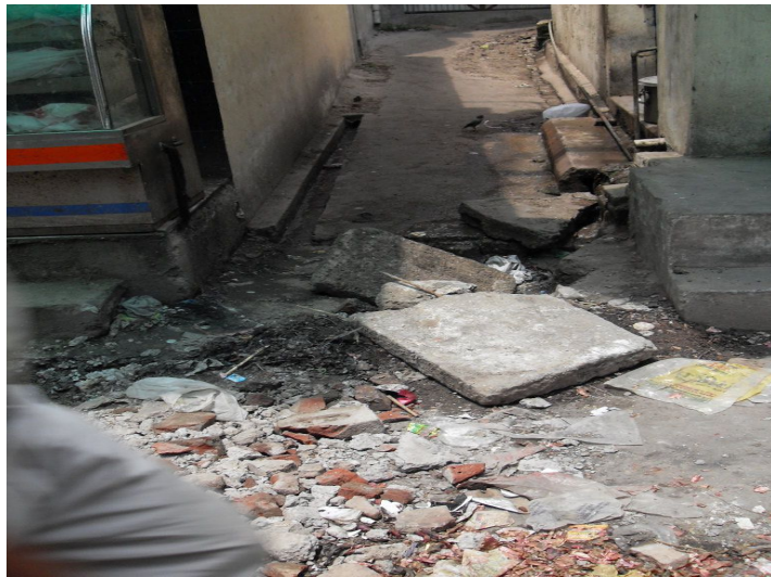
OPEN DRAIN, NO SEWERAGE
