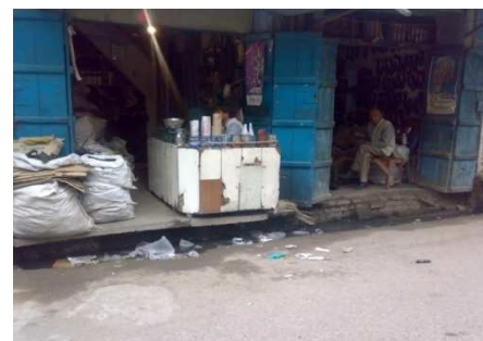
Fig no. 38: Open Drain in Town
