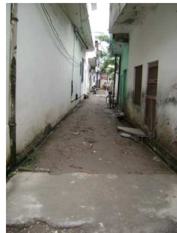
Fig no.24: Open Drains within slum colonies
