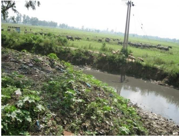
Fig No. 55:- Untreated sewage effluent carried by Nabipur cut drain at crossing section of NH-15 Amritsar
