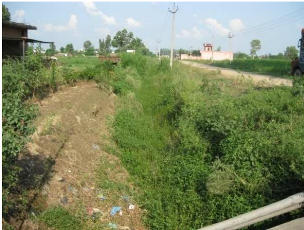
Fig No. 53:- Distributory is full of weeds, shrubs & domestic refuses instead of water supply at Trimu Road
