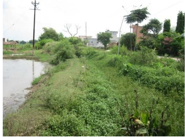
Fig No. 52:- Distributory is full of weeds, shrubs and domestic refuses instead of water supply near ITI Institute
