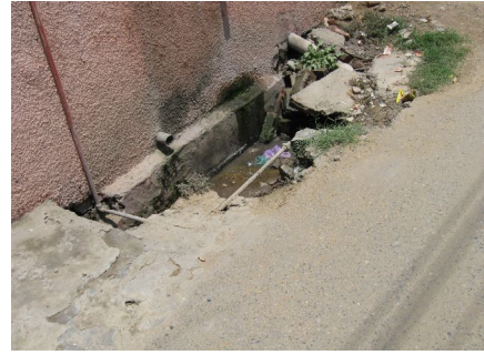
Fig no.36: Open drain along road
