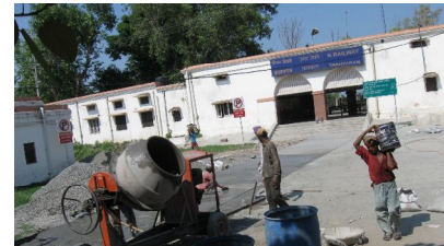
Fig no. 35: View of Railway Station
