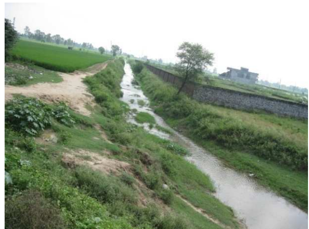
Fig No.58:- Upstream (at Tibri Road, near bridge) of drain has relatively lower pollution level than downstream
