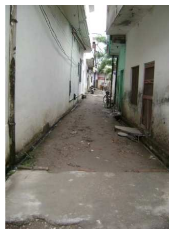
Fig no.24: Open Drains within slum colonies
